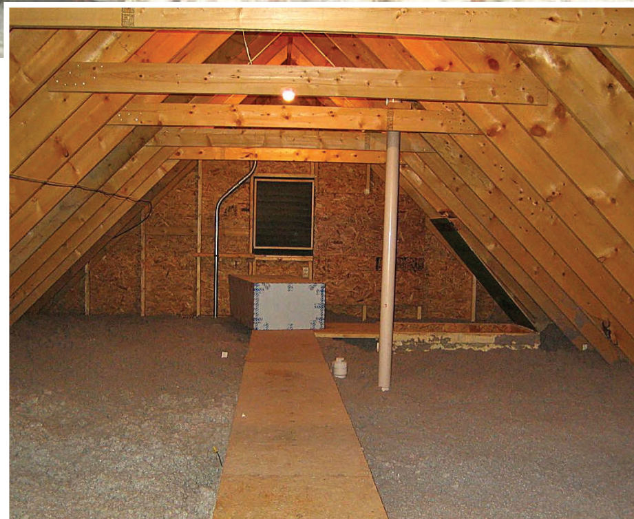
Preventing energy loss. Home Innovation Research Labs is developing solutions for insulation in existing homes' attics with cathedral ceilings, habitable space or those used for storage.
