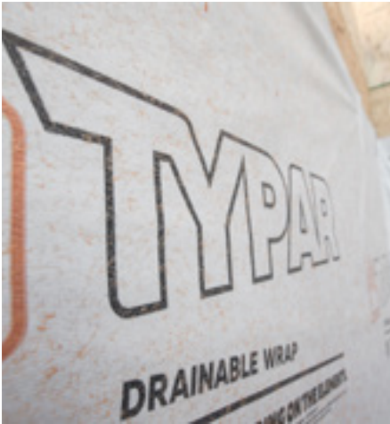
Figure 2. Building wraps made of polyethylene or polypropylene fabric have been a popular method of protecting homes and buildings against moisture intrusion since the 1970s.
