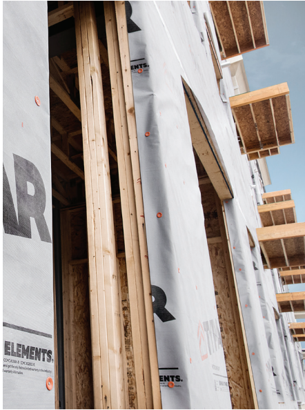
Figure 1. TYPAR Commercial in use on a multi-family building.
