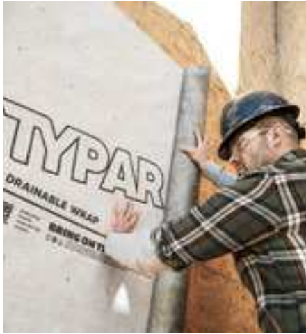
Figure 3. The American Architectural Manufacturers Association defines WRBs as a surface or a wall responsible for preventing air and water infiltration to the building interior.
